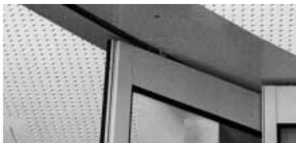
View from below: Track and drive assembly integrated in the suspended ceiling
