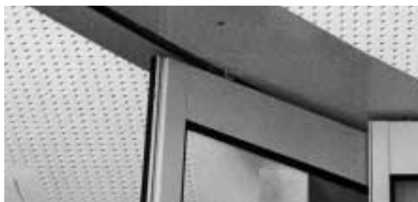
View from below: Track and drive assembly integrated in the suspended ceiling
